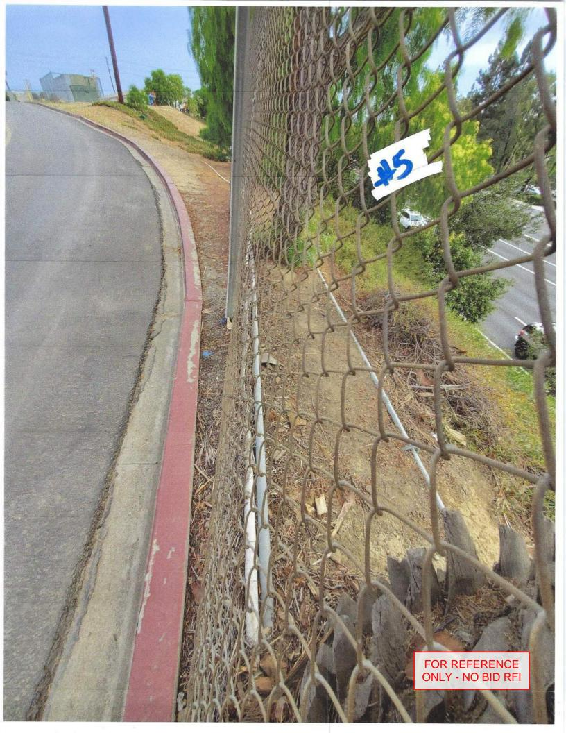
BIDDER RESPONSIBLE TO MAKE REASONABLE EFFORT TO MOVE SURFACE-LAID PIPING/CONDUIT OUT OF THE WAY OF NEW WORK, INCLUDING POSSIBLE TEMPORARY RAISING AT PALM TREE.
